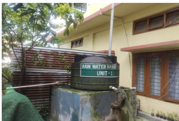
Rain water harvesting unit
